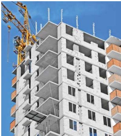
Perimeter walls in precast building
