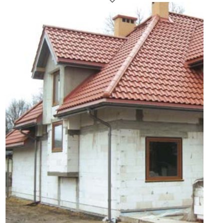
Load bearing walls in family houses
